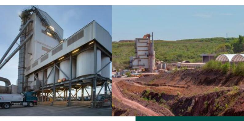
2023. They keep the materials dry, meaning less gas is needed to heat them when used in the mixing process.
